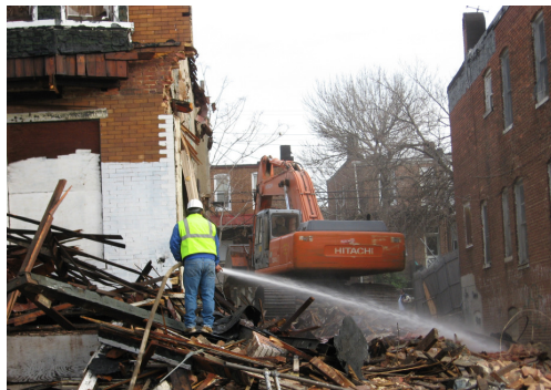
2731 Tivoli Ave. after demolition
